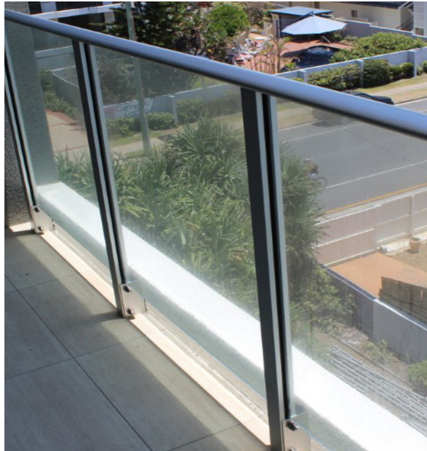
Glass balustrade with metal handrail
